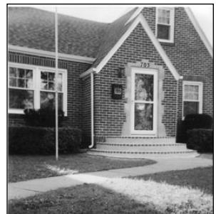
Bahm's Complete Concrete Face lift for your concrete
